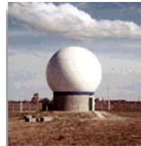
ORBCOMM Earth Station
